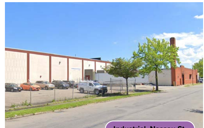
Industrial, Nassau St.
