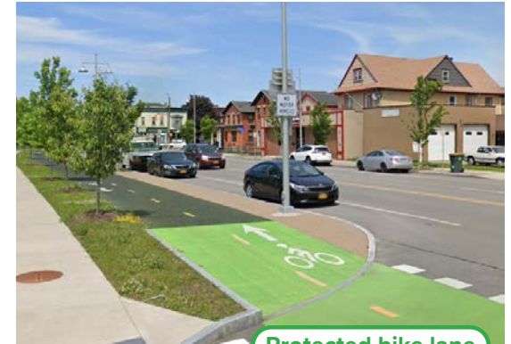
Protected bike lane
