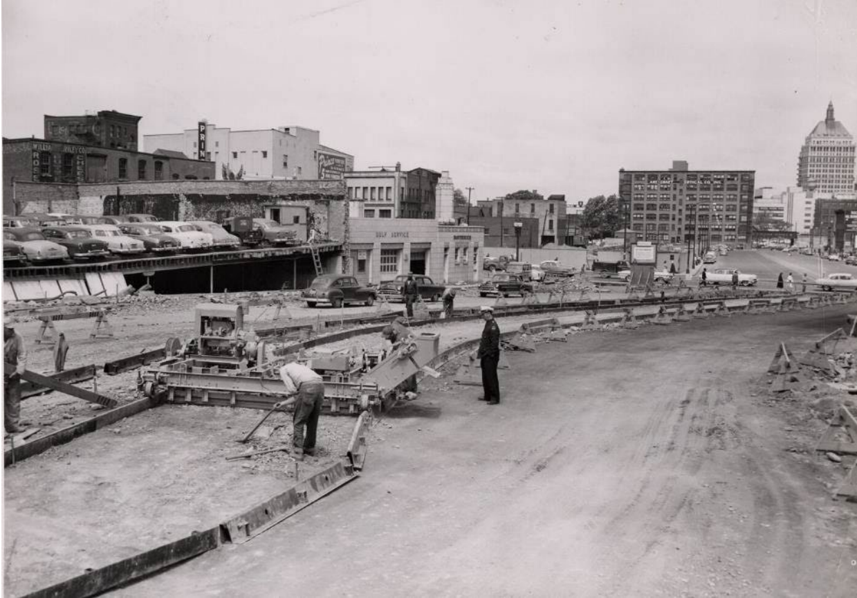
Construction of the Inner Loop in 1957, with Kodak Tower in the background. Photo credit: Ernest Amato, from the Collection of the Local History and Genealogy Division, Rochester Public Library
